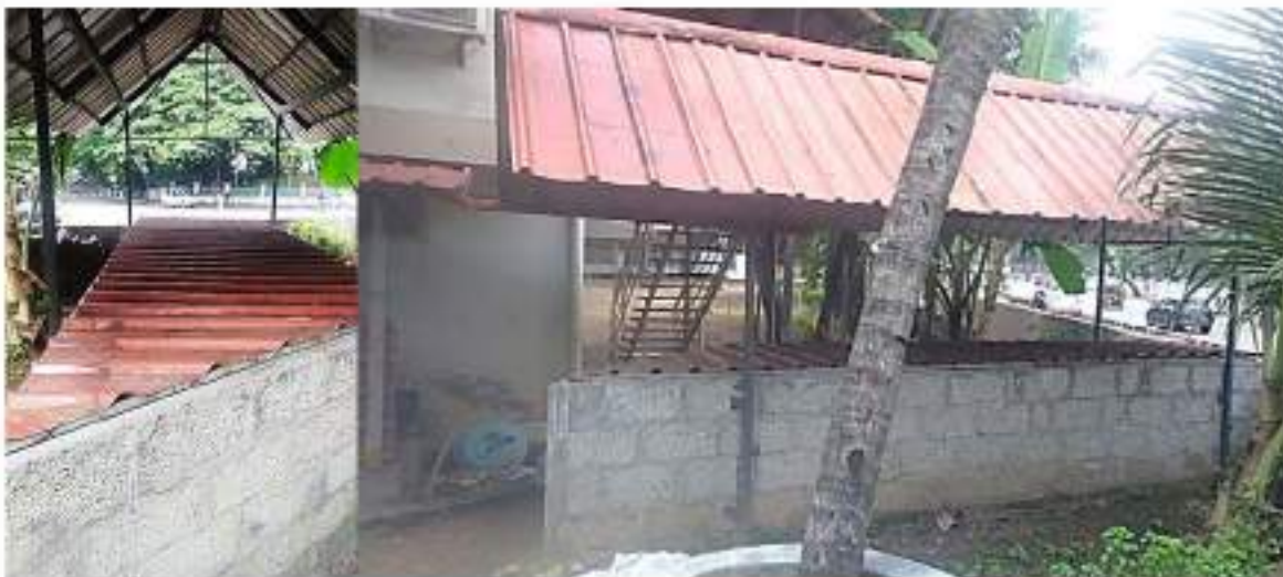
Composting unit established in the church campus (A tank is divided into two units)
